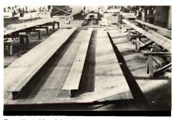
Figure 46 Vail Pass Colorado Bridges: bottom flange stiffeners.
