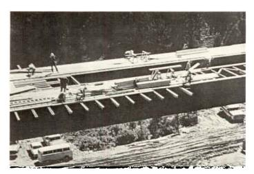
**Figure 59** Vail Pass Colorado Bridges: formwork for concrete deck slab.
