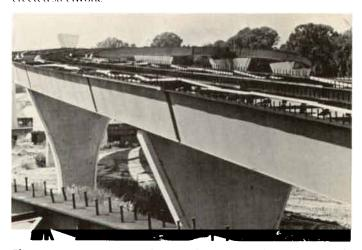
**Figure 64** Louisiana Airline Highway Interchange: erected steelwork.
