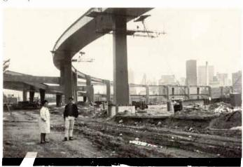
**Figure 73** Pittsburgh's Fort Duquesne Bridges: erection of curved-box sections.
