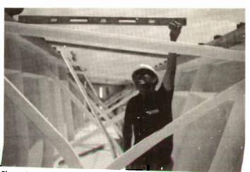
Figure 81 Twist of Girder.
