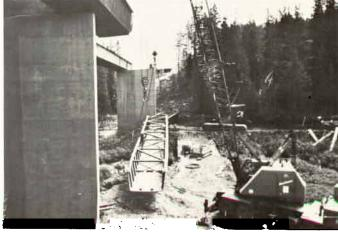
Figure 52 Vail Pass Colorado Bridges: erection of shipping piece.
