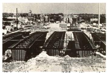
**Figure 79** Erected Girders Prior to Distortion.
