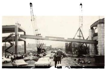
**Figure 72** Pittsburgh's Fort Duquesne Bridges: erection of box-girder span to bents.
