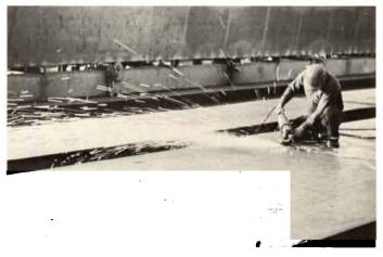
Figure 45 Vail Pass Colorado Bridges: bottom flange preparation.
