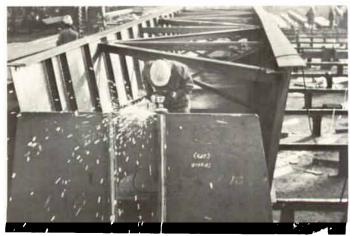
Figure 49 Vail Pass Colorado Bridges: end diaphragm fabrication.
