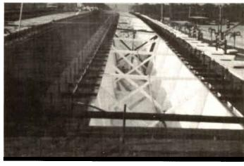
Figure 80 Bowing of Girder.
