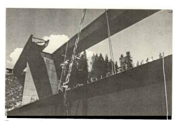
Figure 54 Vail Pass Colorado Bridges: erection of shipping piece.
