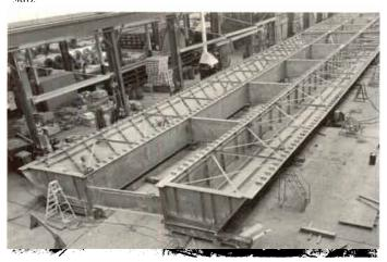
**Figure 60** Omaha Nebraska Viaduct: shop assembly showing crossframe lateral bracing arrangement.
