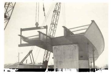
**Figure 61** Omaha Nebraska Viaduct: erection of curved-box section.
