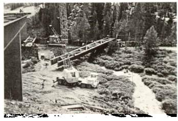
Figure 51 Vail Pass Colorado Bridges: erection of shipping piece.
