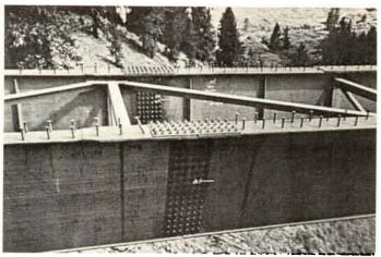
**Figure 56** Vail Pass Colorado Bridges: field splice and flange transition.
