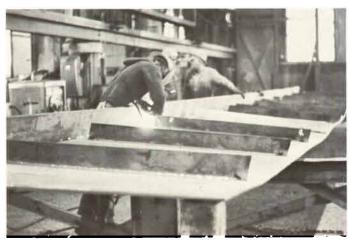
**Figure 47** Vail Pass Colorado Bridges: web to top flange fabrication.
