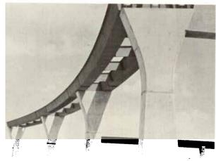
**Figure 66** Louisiana Airline Highway Interchange: erected sections of curved-box girders.
