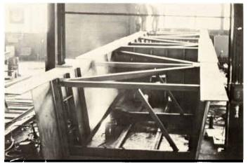
**Figure 44** Vail Pass Colorado Bridges: crossframes and lateral bracing arrangement.
