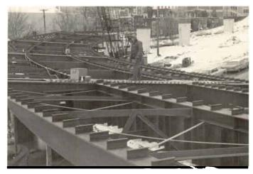
**Figure 62** Omaha Nebraska Viaduct: erection of curved-box sections.
