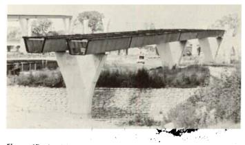
**Figure 67** Louisiana Airline Highway Interchange: erected sections of straight-box girders.
